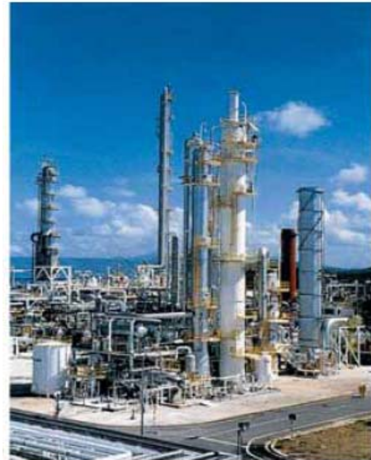
↑ CO_2 capture by chemical absorption (fertilizer plant in Malaysia)
