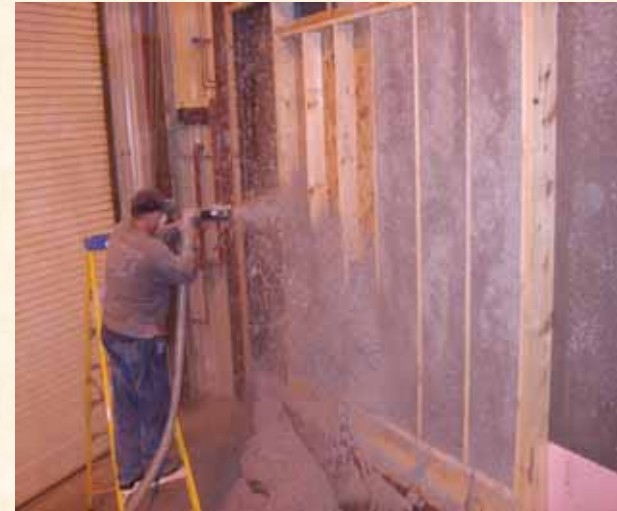
Installation of PCM-enhanced cellulose insulation in a test wall
