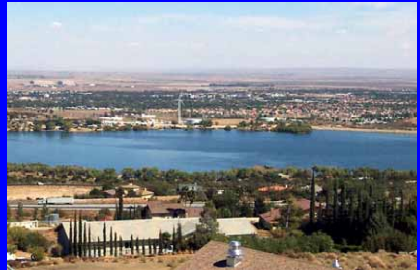
The Palmdale, CA Treatment Plant
