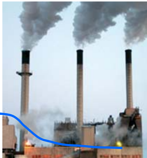
Figure 1: 220 MW, coal-fired power plant in Vailmont, Colorado, where tunable diode laser measurements of gas temperature were made. Successful measurements were made with less than 1% optical transmission.
