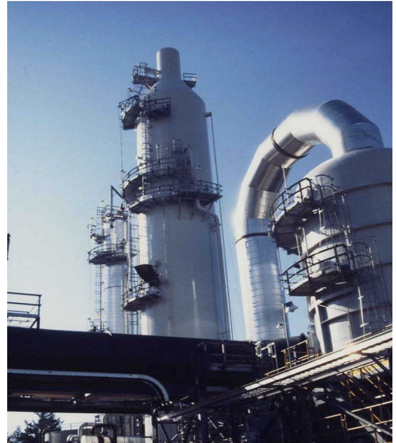
ECONAMINE™ Unit at Bellingham, MA CO 2 Plant Courtesy of Val Francuz (Fluor) and Cliff Lowe (CVX)
