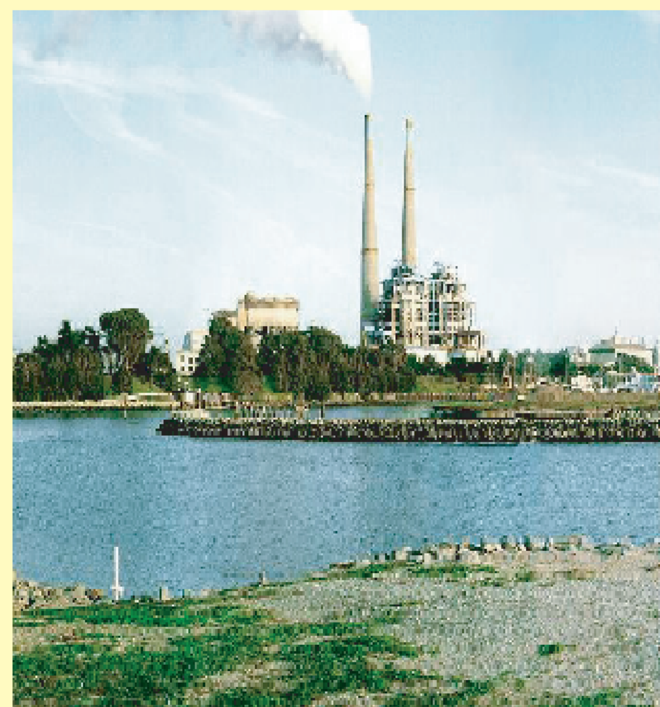
A coastal NG-fired power plant Moss Landing, CA - candidate for wet limestone scrubbing.
