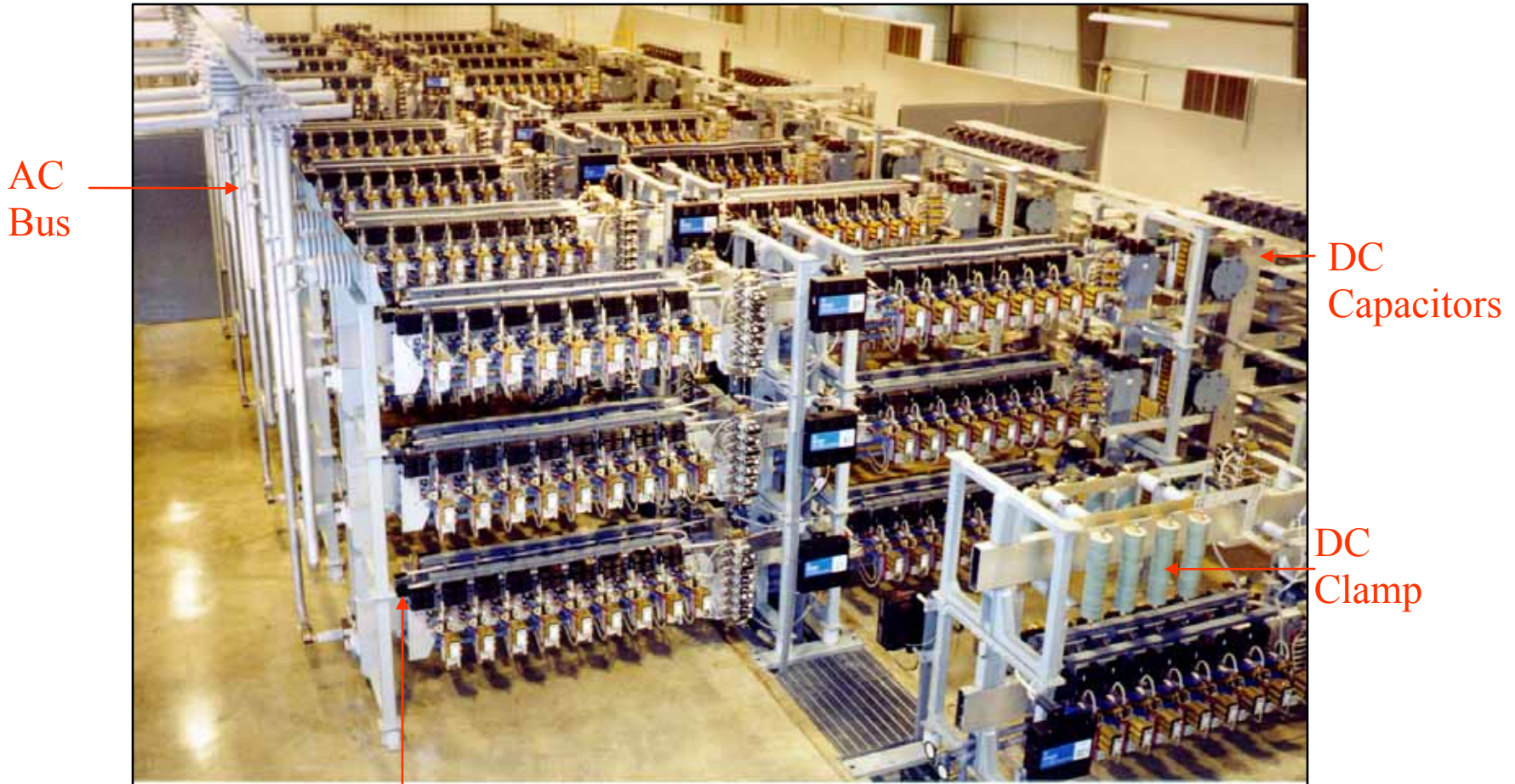
Inverter Pole Assembly
